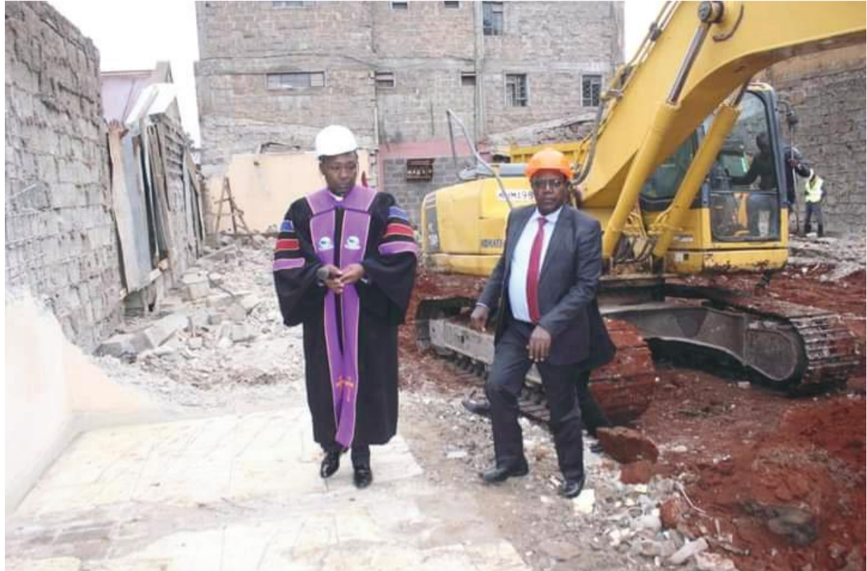
Biashara Sacco chairman Joseph Njamuku with Bishop Paul Wanjohi embarks from one of the equipment that will be used during the construction of the complex. Photo/PAUL MWANGI WANJIRU.
