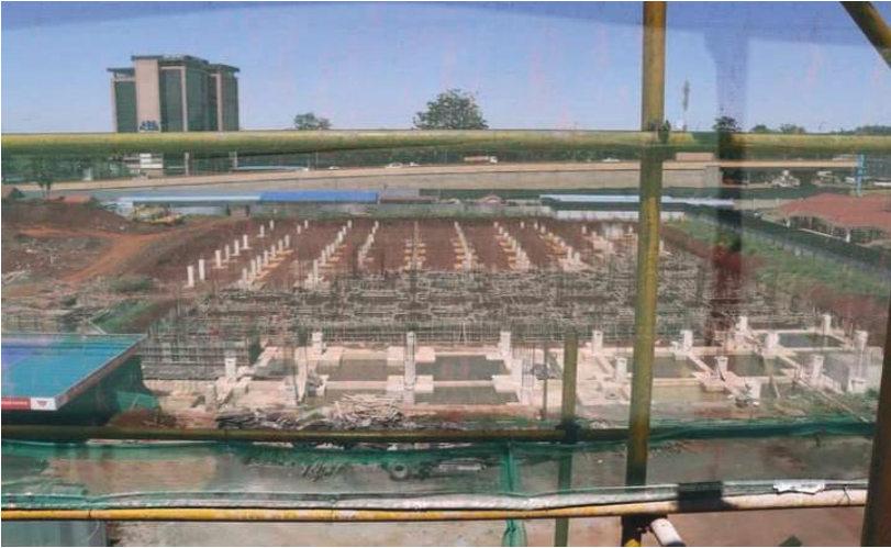
Part of the facility under construction.
