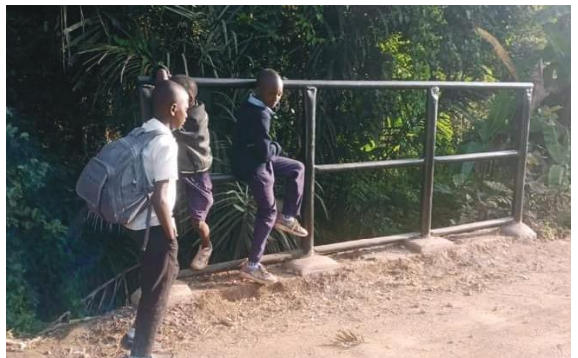
Mboone River Bridge In Igembe Gets Barrier Rails To Enhance Safety.
