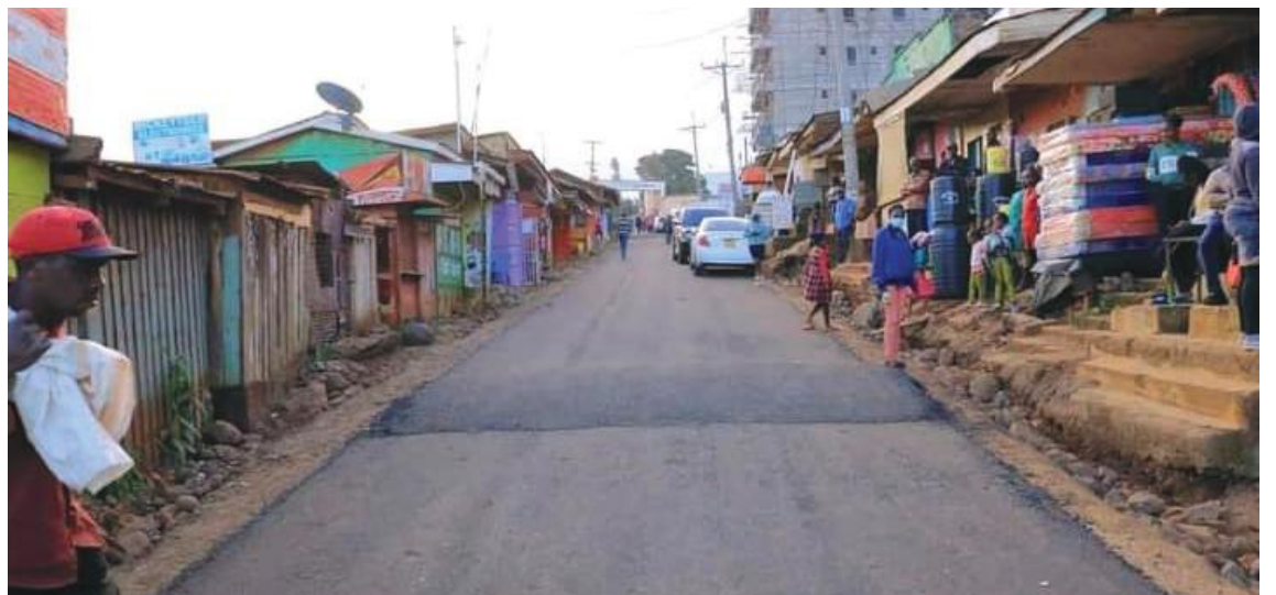
Roads in a rural town being rehabilitated
