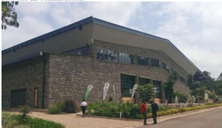
The modern Jamhuri Park Exposition and Conferencing Center which was constructed with funding from the national government and the Agricultural Society of Kenya (ASK) and was completed in 2022. Photo by Joseph Ng'ang'a.
