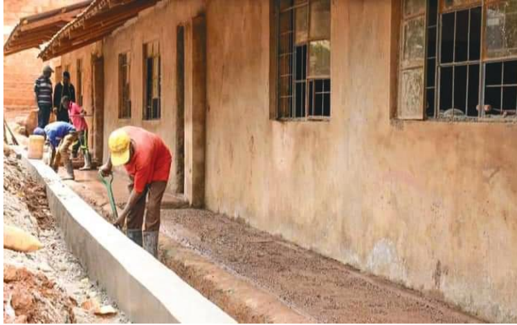
One of the school undergoing face-lift in Kangema constituency.
