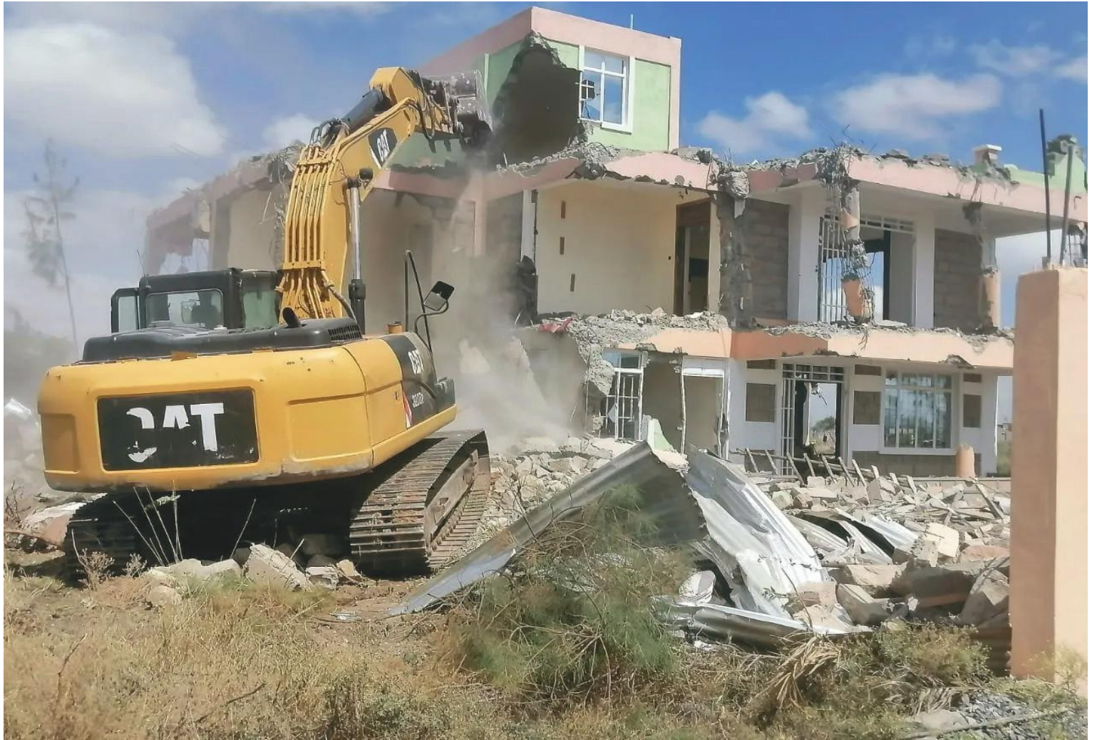
Athi River Demolitions.
