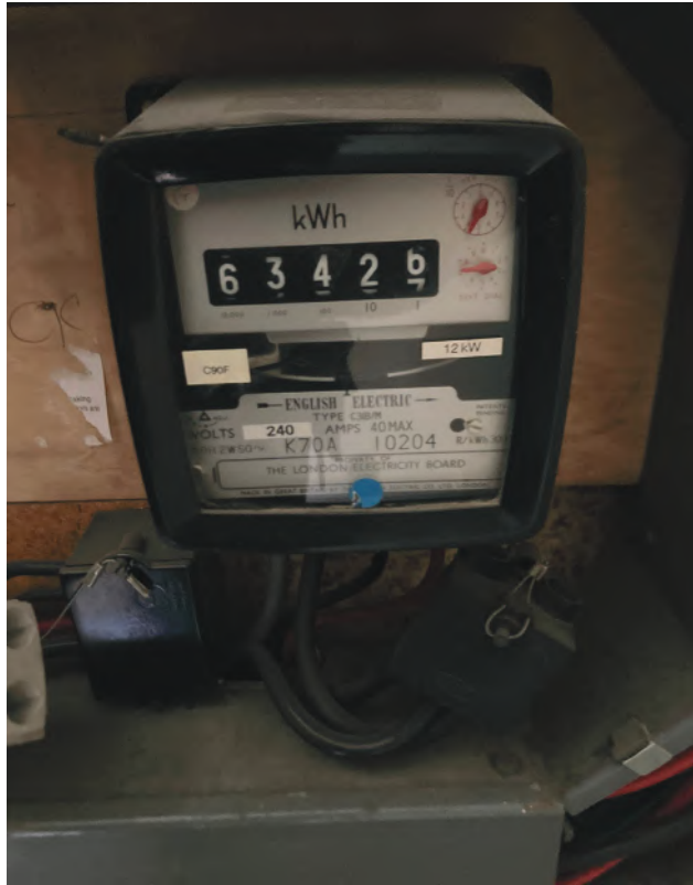
Crippling costs of energy are taking a toll on families who avoid heating their homes, Photo SHAMLAL PURI
