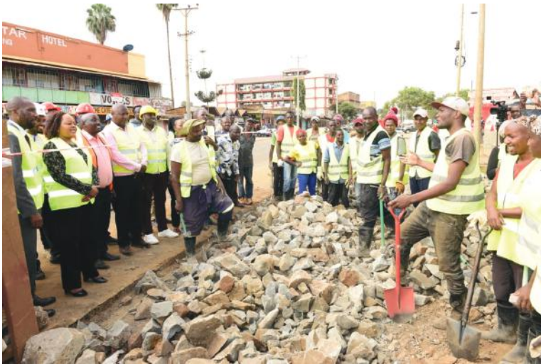
Kirinyaga County Governor Anne Waiguru during an inspection tour of Sagana Cabro project.
