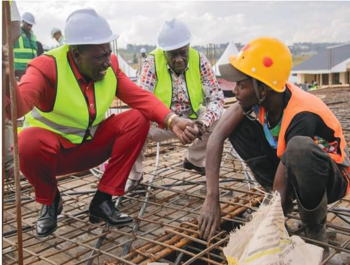
President William Ruto (left), his deputy Rigathi Gachagua (center) listens as a worker explain how they are undertaking Affordable Housing project in Ol-Kalou, Nyandarua County..
