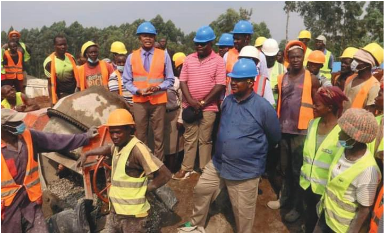
Leaders at one of the Affordable Housing construction sites..
