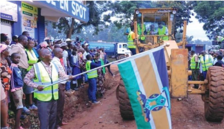
Rehabilitation of one of the roads being launched
