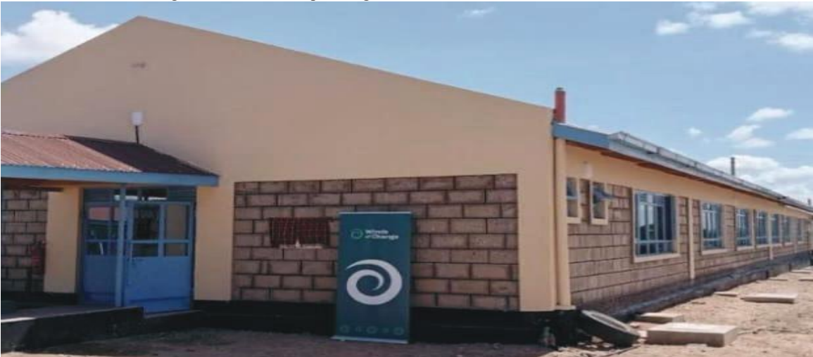
A 22-bed capacity male ward constructed by LTWP at the Laisamis Sub-County Hospital at a cost of KSh15.3 million under its corporate social responsibility programme, the Wind of Change.
