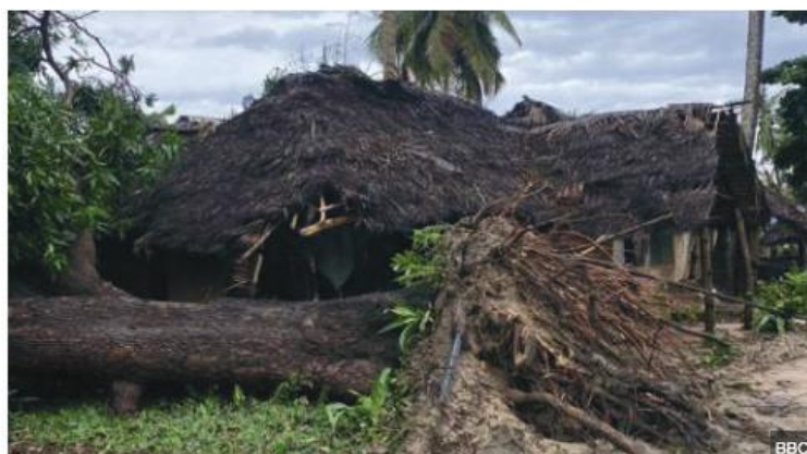
A house destroyed in Mafia Island as a result of Cyclone Hidaya
