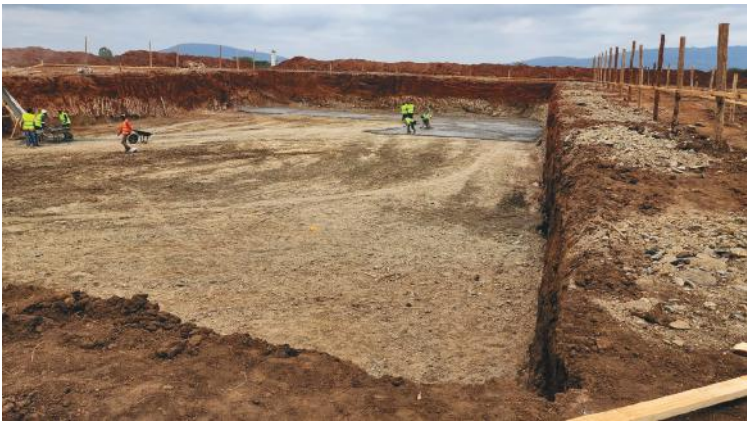
Construction of an Olympic-standard aquatic sporting facility ongoing in Machakos town
