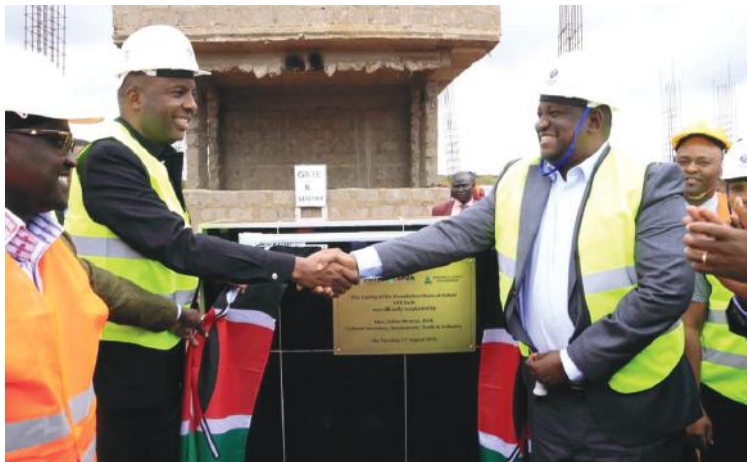
Trade CS Salim Mvurya and Murang'a Governor Irung'u Kangata, during the launch of the construction of the first phase of Kabati (Mitumbili - Gatanga) Export Processing Zone (EPZ) in Murang'a County..
