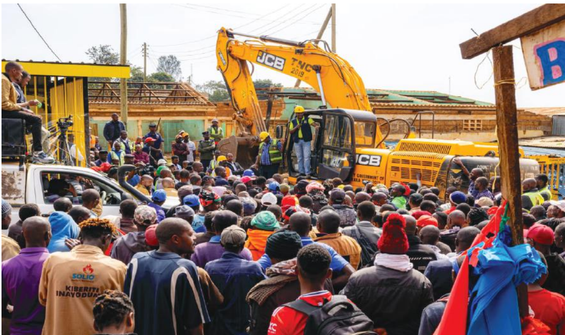
Chuka market demolition
