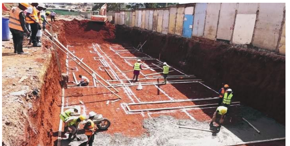
The new Embu market under construction
