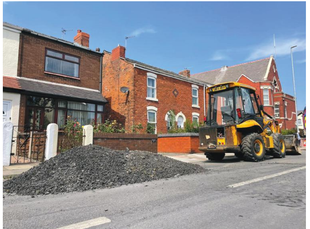
The morning after the days of violence, rebuilding works start in Southport.
