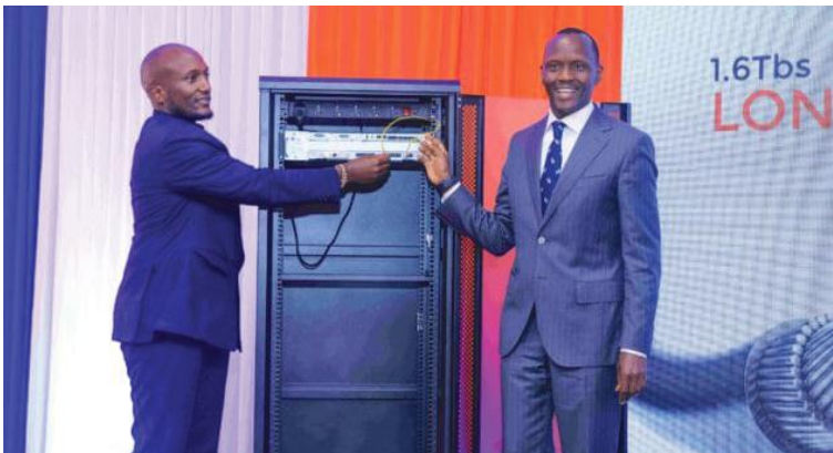
Syokinet Solutions CEO, Ian Kasyoki, (left) and KPC MD, Joe Sang (Right) officiate the onboarding of Syokinet Solutions to KPC's fibre optic cables network.
