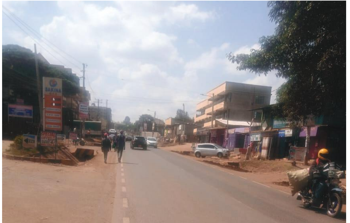
The black spot Kiambu town road where seven lives were lost through road accident in the past one month due to lack of rumble bumps
