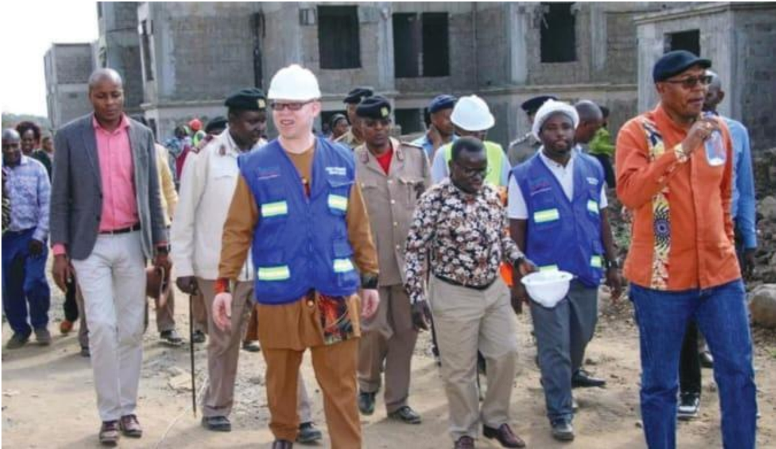
Government Spokesperson, Isaac Mwaura, leads a team to inspect construction of Affordable Housing at Makenji in Murang’a..
