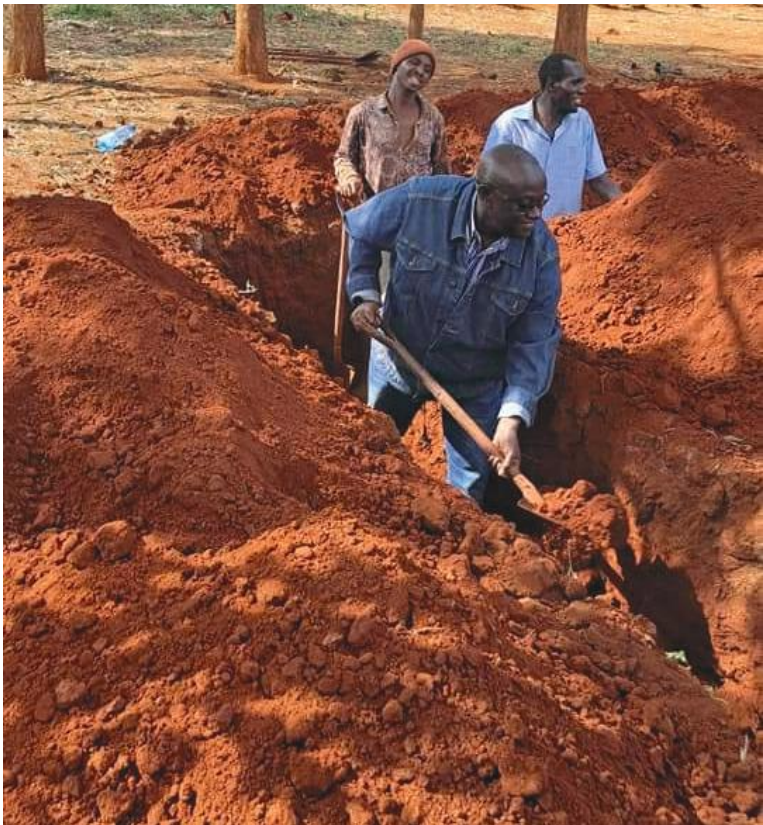
Lawrence Mwaura Ting'ang'a Ward MCA breaking ground of an ECD center in his ward
