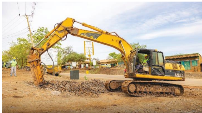
Ongoing construction of roads in Marimanti and Kathwana towns. Photo/Mwenda Njeru.
