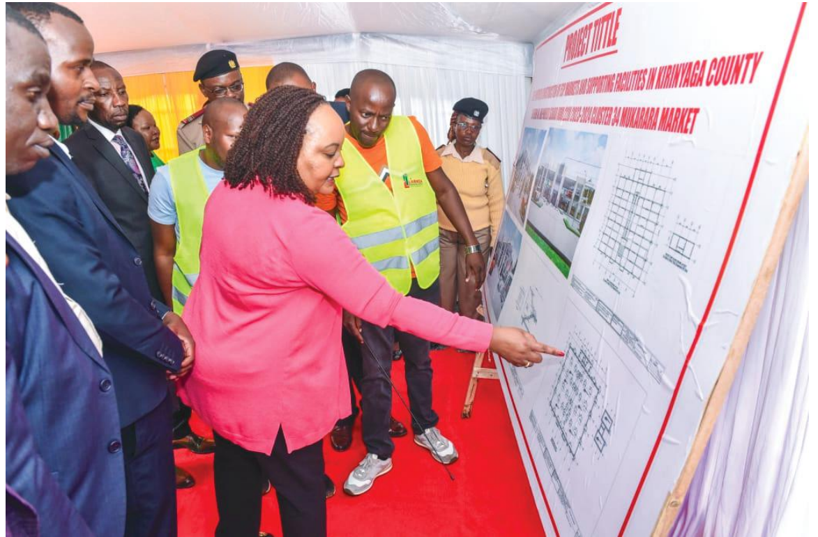
Governor Anne Waiguru with traders at Kagio town in Kirinyaga County ultra-modern market construction site
