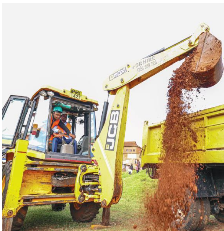
Deputy President Prof Kithure Kindiki groundbreaking the Othaya Stadium.
