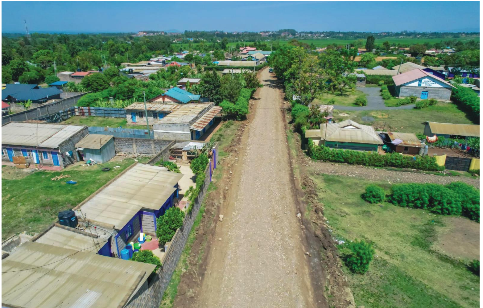
One of the rehabilitated road in Kirinyaga County. Photo/Courtesy.
