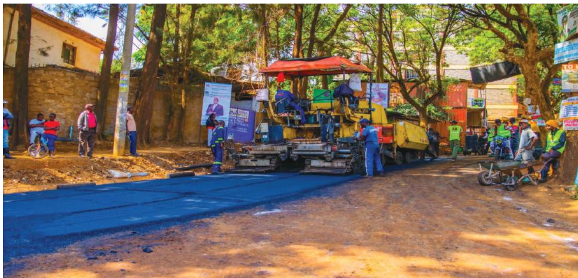
Different roads that are being tarmacked in Kiambu constituency under the Kenya Urban Roads Authority (KURA).
