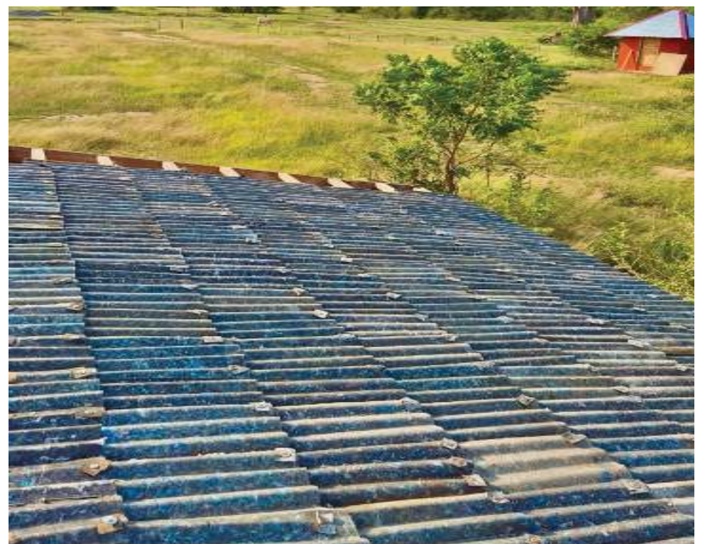
A roof made from plastic waste
