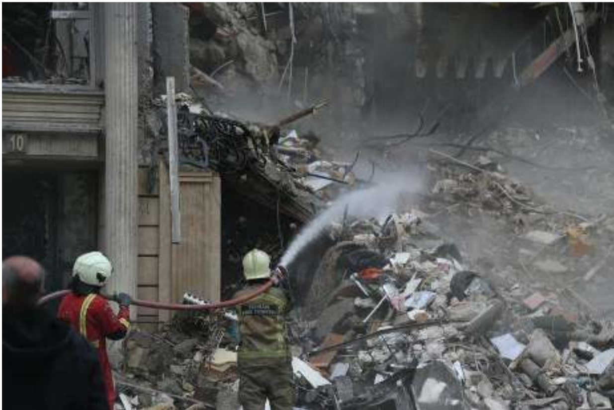
This photo taken on March 23, 2026 shows a destroyed building in a residential area after joint U.S.-Israeli strikes on Iran in Tehran, Iran. | Photo: Xinhua/Shadati
