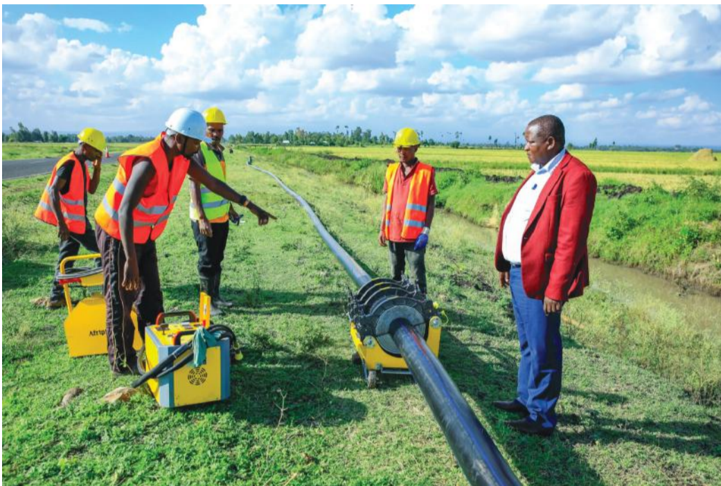
Officials inspecting the works
