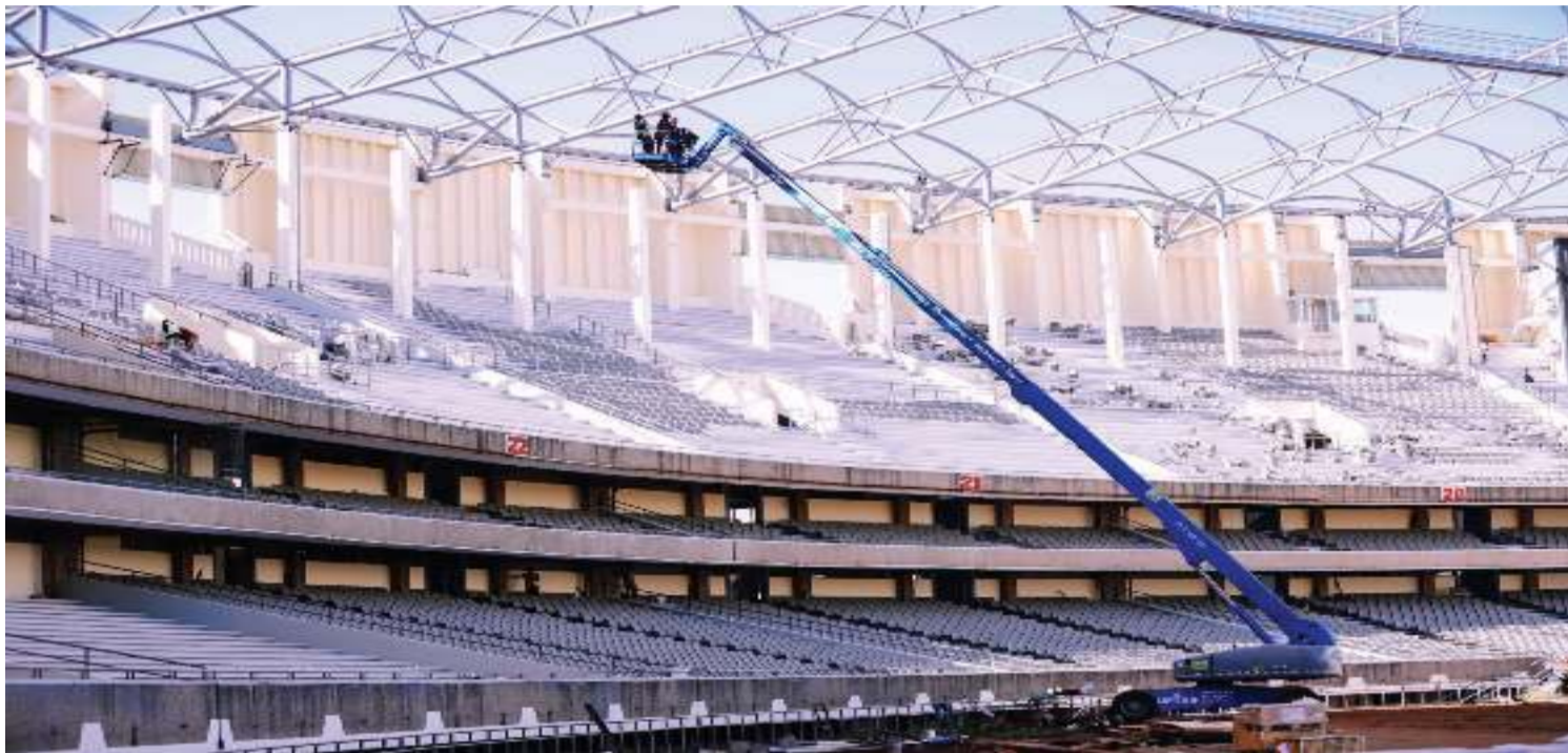
Ongoing works at the Kasarani Stadium. PHOTO/FOOTBALL KENYA FEDERATION
