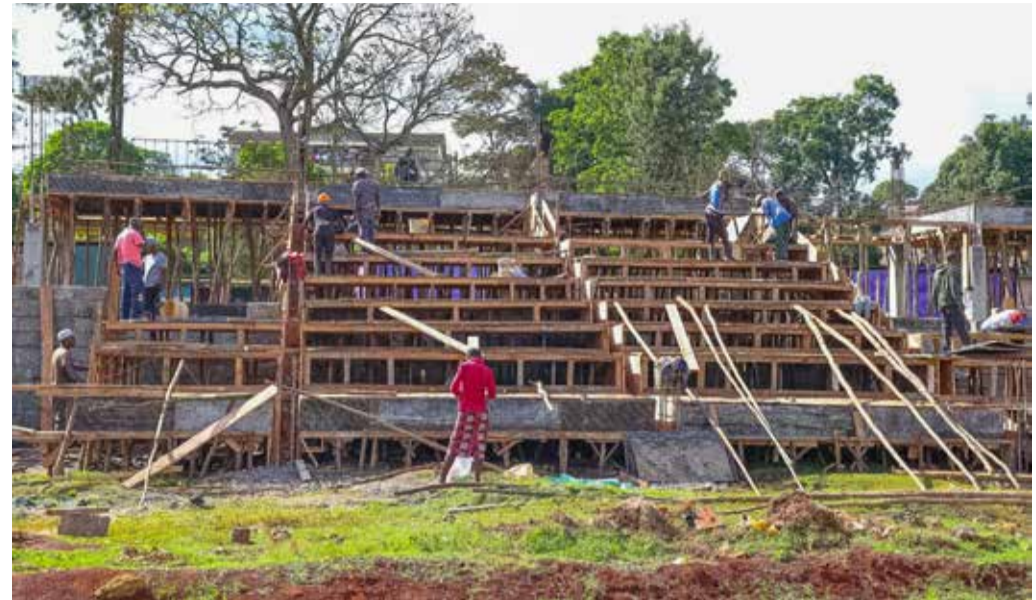
Workers at Othaya stadium yesterday | Photo: Courtesy.
