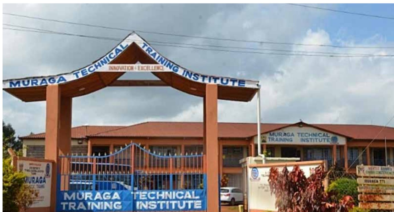
A view of Muraga Technical Training Institute in Tharaka-Nithi County from the main gate. | Photo: Dickson Mwit.
