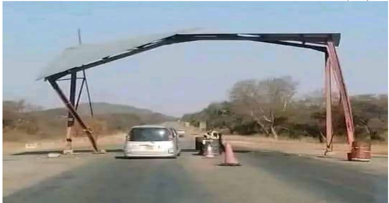
Posh estate entry gate
