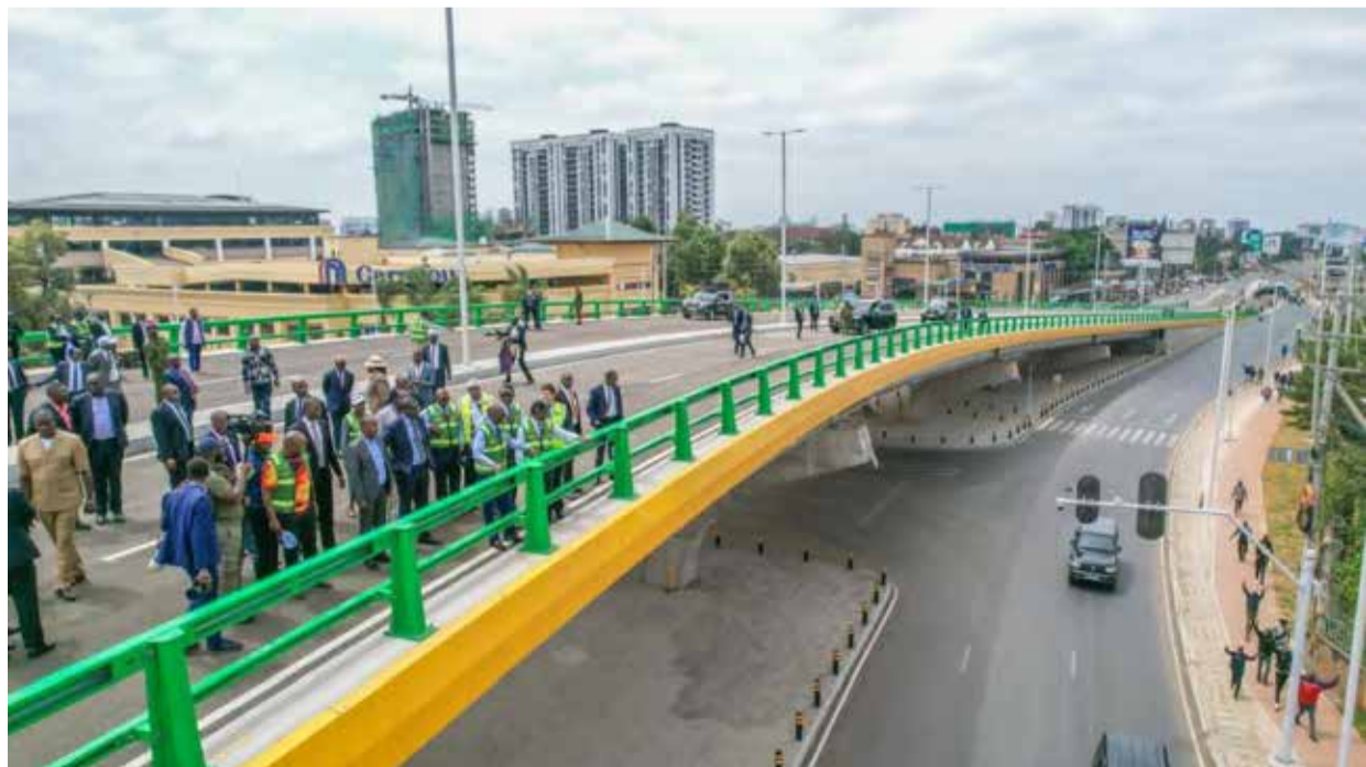
The president and other leaders atop the viaduct.
