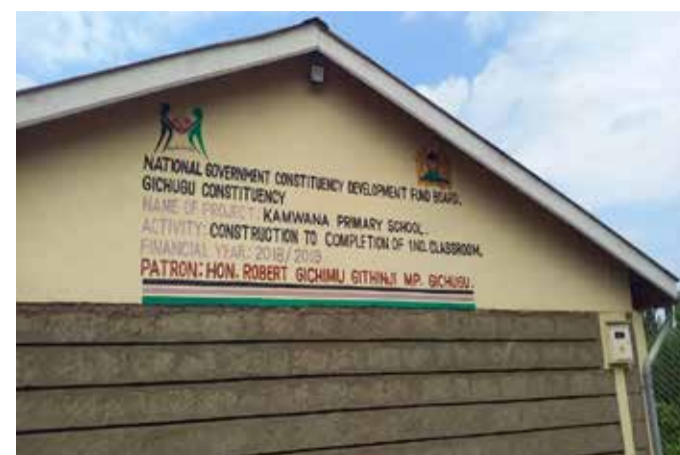
Writing on a wall at the newly built Kamwana Primary school in Gichugu constituency.
