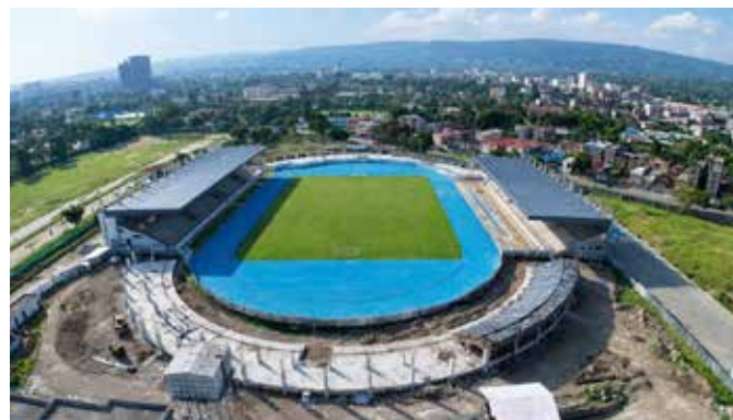
Afraha stadium that is being constructed by KDF. | Photo: Courtesy.
