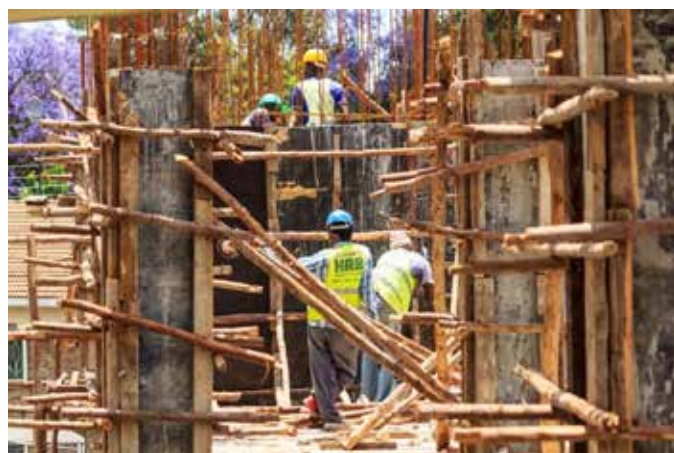
A construction site
