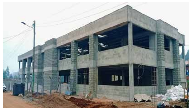
Part of Ndungu SP market that is under construction
