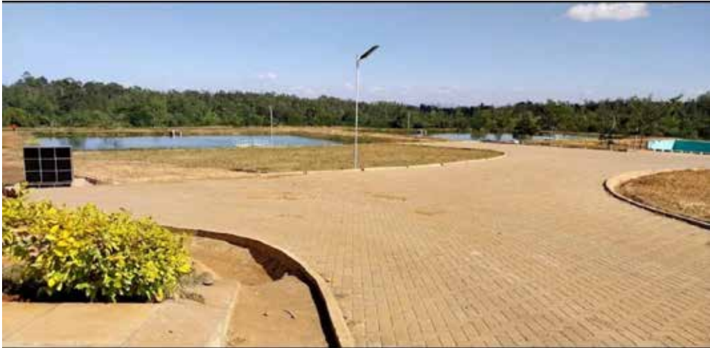
Chuka Sewage system in Tharaka Nithi County| Photo: Alex Njeru.
