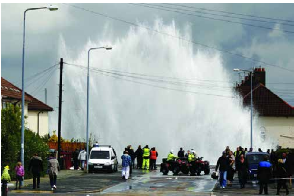
Large diameter burst water mains such as this in Liverpool caused a lot of losses and water shortages, adding to the headache of Britons. Photo Courtesy
