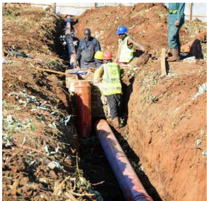
Construction works continue at the new temporary market site at Gakoromone. | Photo: Brian Gitonga
