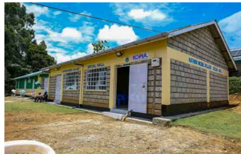
Potato storage facility and social hall. | Photo: Brian Gitonga
