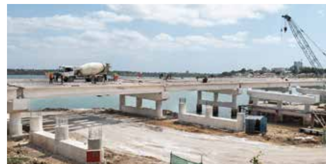
Bamburi Cement Makupa Bridge concrete. | Photo: Courtesy
