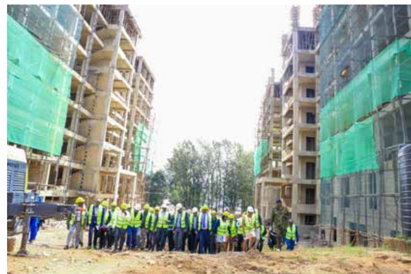
Nyanchwa Affordable Housing Project in progress. | Photo: Elizabeth Angira
